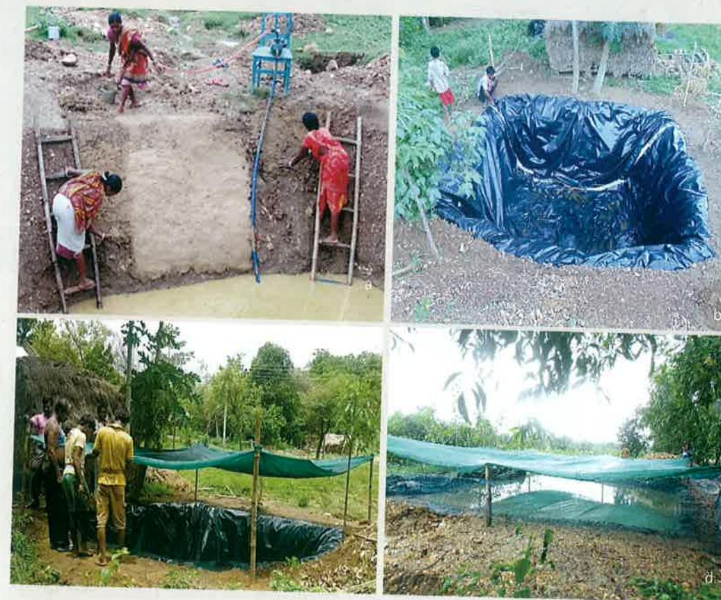
Fig. 2: Rain water harvesting programme in Bhutadhi village of Purulia. Here polythene sheet layered small ponds (poly-pond) were constructed for collecting rain water for irrigation purpose. The scheduled tribe beneficiaries were preparing their own reservoirs under Bose Institute's guidance. Purulia district of West Bengal is a low rain fall area
