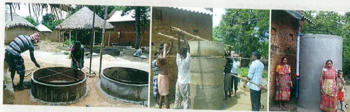
Fig. 1a-1c: Rain water harvesting programme in Bhutadhi village of Purulia. Here concrete reservoirs (2,000 L capacity) were constructed for collecting rain water for drinking purpose. The scheduled tribe beneficiaries were constructing their own reservoirs under Bose Institute's guidance. Total 16 Nos. of tanks have been constructed so far in Bhutadhi village (13Nos) of Purulia and Chhachanpur village (3Nos) of Bankura.
