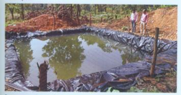
Representative poly-pond at Amlasole (size of this pond is 22'x20'x7', capacity ~75,000 L). Fifteen such poly-ponds were constructed so far in Purulia and Pashchim Medinipur for harvesting rain water. Demonstrations are being given in these regions for utilization of this water for watering orchard plants, vegetables cultivation, cultivation of low water requiring crop plants and toilet use.
